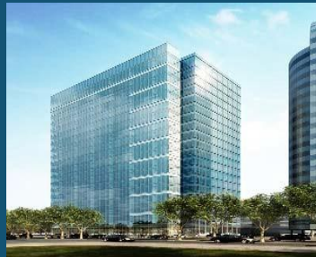
Millennium Tower II
